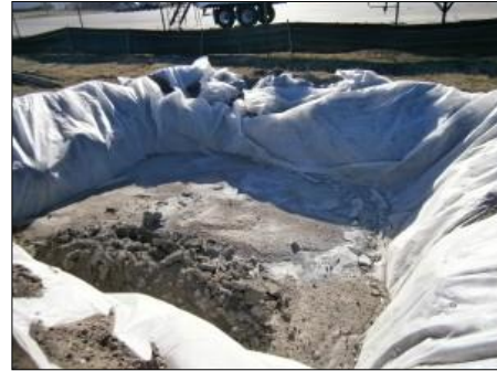
Plate 4-2 Concrete washout area
