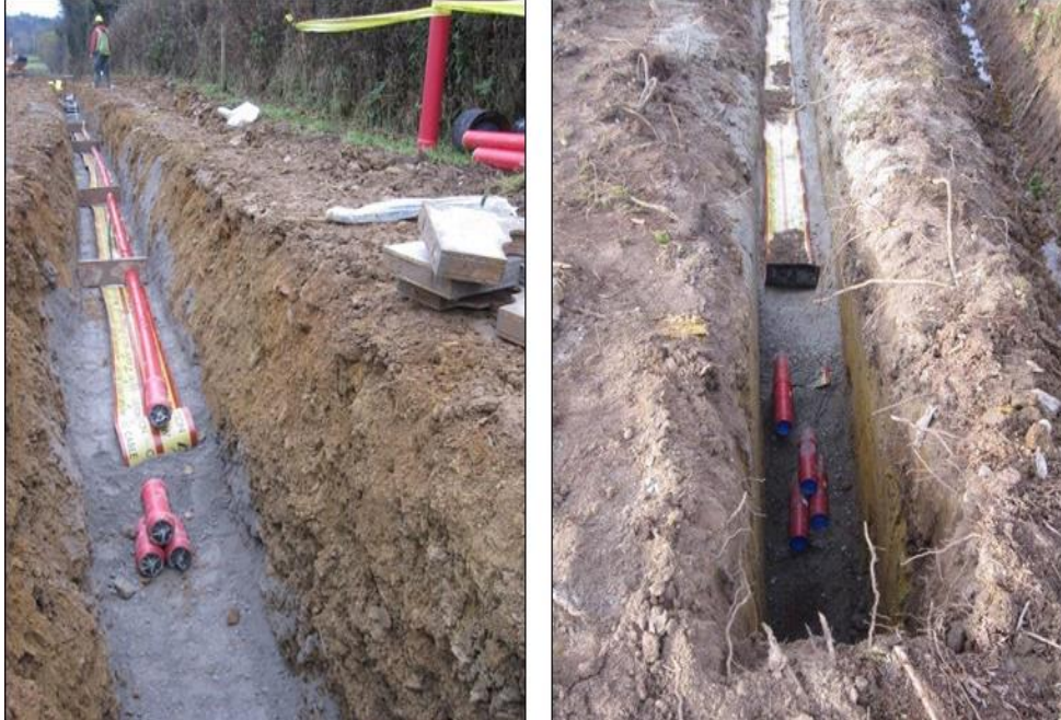
Plate 4-5 Typical Cable Trench View
