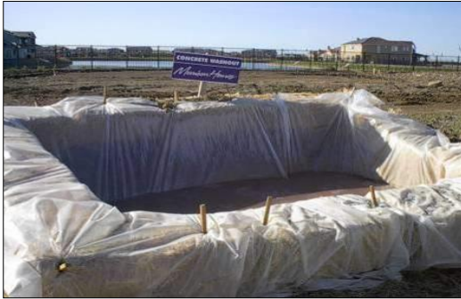
Plate 4-1 Concrete washout area
